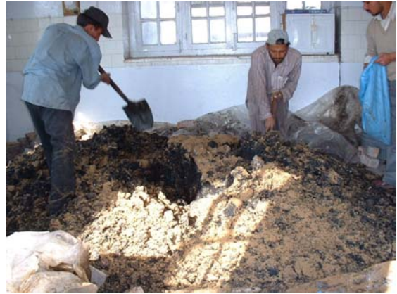
Mixing of Bokashi in Sludge
